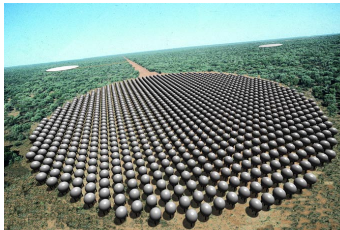
Figure 2 - Artist's impression of an SKA station using 5m diameter Luneburg Lenses
