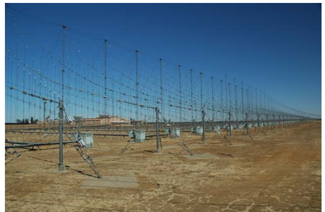
Figure 4. View of the transmitter array at Longreach.
